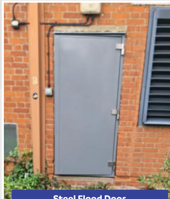
Steel Flood Door (SR2 Security Rated)
