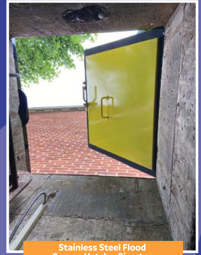
Stainless Steel Flood Escape Hatch – Bicester
