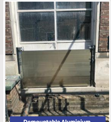
Demountable Aluminium Flood Barrier
