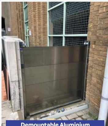
Demountable Aluminium Flood Barrier
